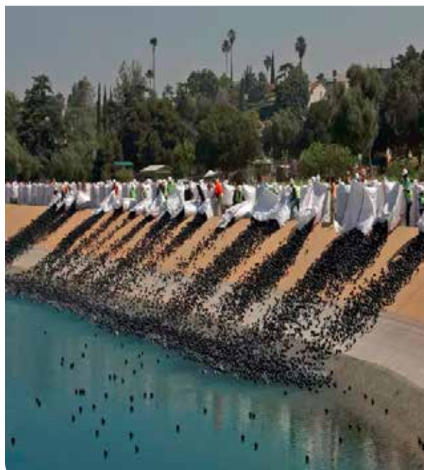
• Reservoirs with thousands of Black Balls In an Effort to reduce Evaporation.
