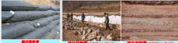
梯田筑软埂 soft ridge construction in terraced field
