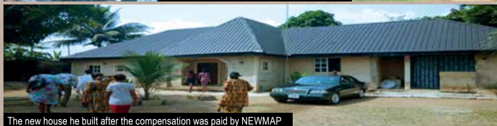
Project Beneficiary whose house was affected by gully erosion and was paid compensation
