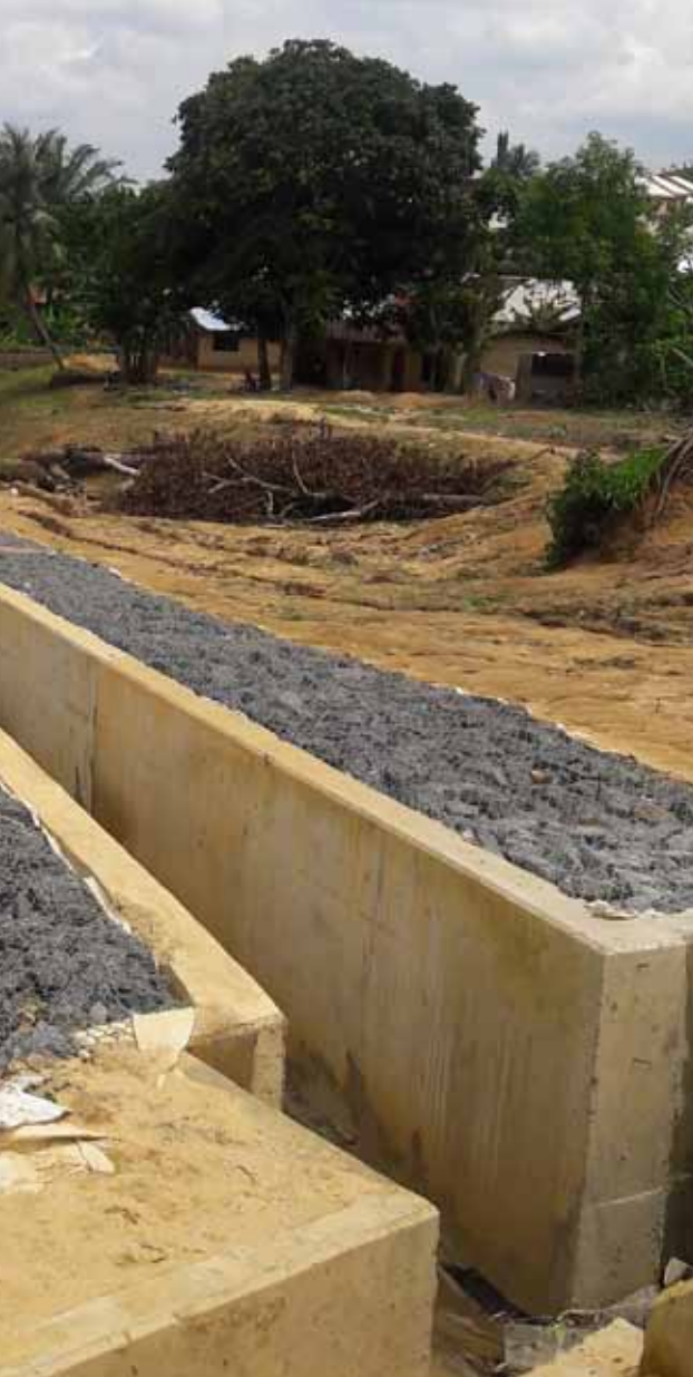
Properly terminated drainage in finger 2 Ikot Anwatin site, Cross River State.
