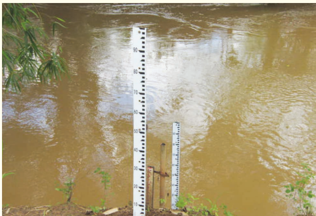
Installed manual River gauges in Itu LGA of CRBDA
