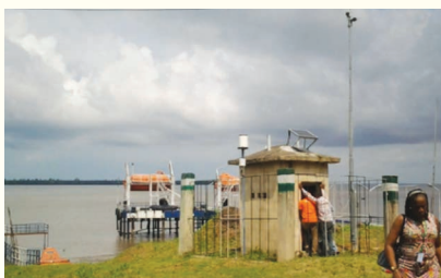
Installed Automatic Flood Early Warning System (AFEWS) in Oron, CRBDA
