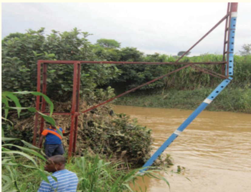
Typical sensor for automatic hydrological stations
